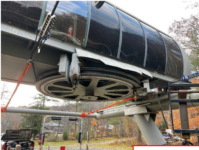
Bullwheel and Haul Rope Rigging
