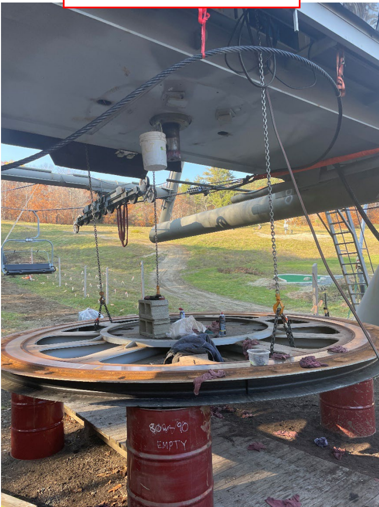
Bullwheel and Haul Rope Rigging
