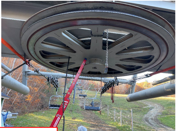
Bullwheel and Haul Rope Rigging
